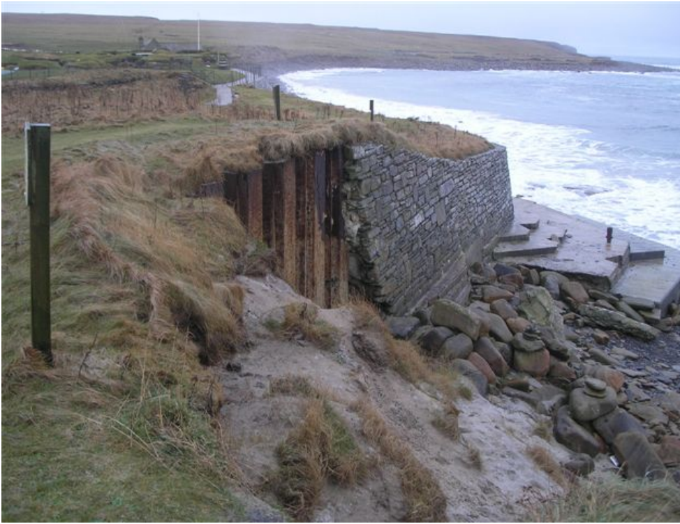
Figure 6 : . Engineered coastal protection of the Neolithic settlement at Skara Brae in Orkney showing damage following winter storms (Image: Historic Scotland)
