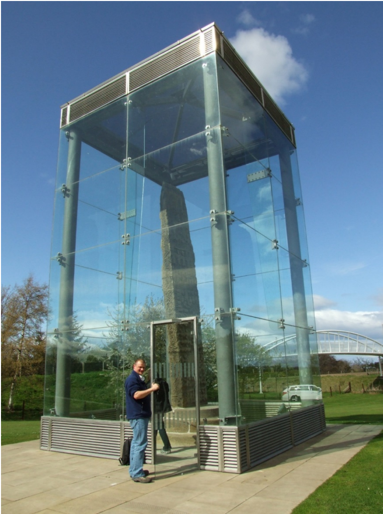
Figure 5 : Protection of a standing stone (Sueno's Stone, Moray) using a naturally ventilated glass structure in order to prevent further deterioration of fragile carved surfaces from rainwater and wind erosion (Image: Historic Scotland)
